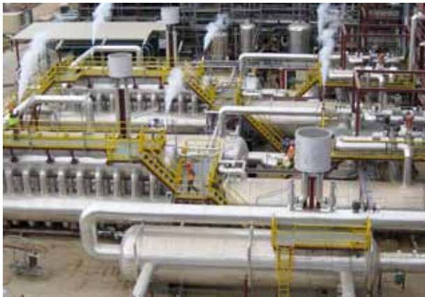
Fig. 8: 2 x 25MWe steam generator line
